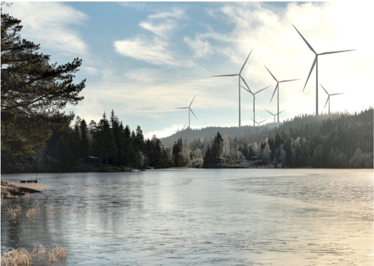
Odal Vind, Odal, Norway
